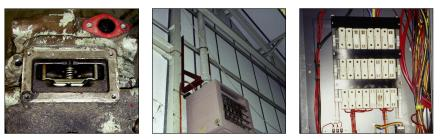
Asbestos isn't always obvious. Would you spot an asbestos gasket on an old engine, asbestos cement pipes or an asbestos-containing fuse-board? If you're not sure, the premises owner needs to get it checked out!
